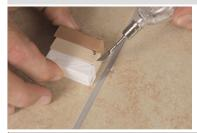
A very hard filler designed to repair scratches, holes and edge damage on ceramic wall and floor tiles. Suitable for use in interior and exterior areas. Melt and fill then level with the Special Ceramic Filler Applicator.
